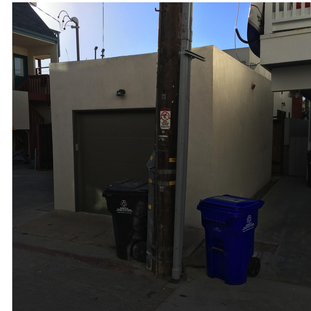
NORTH WEST VIEW
